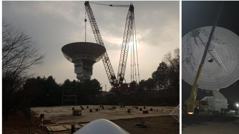
Fig. 3. KDSA 35-meter Main Reflector Lifting and Surface Roughness Measurement
