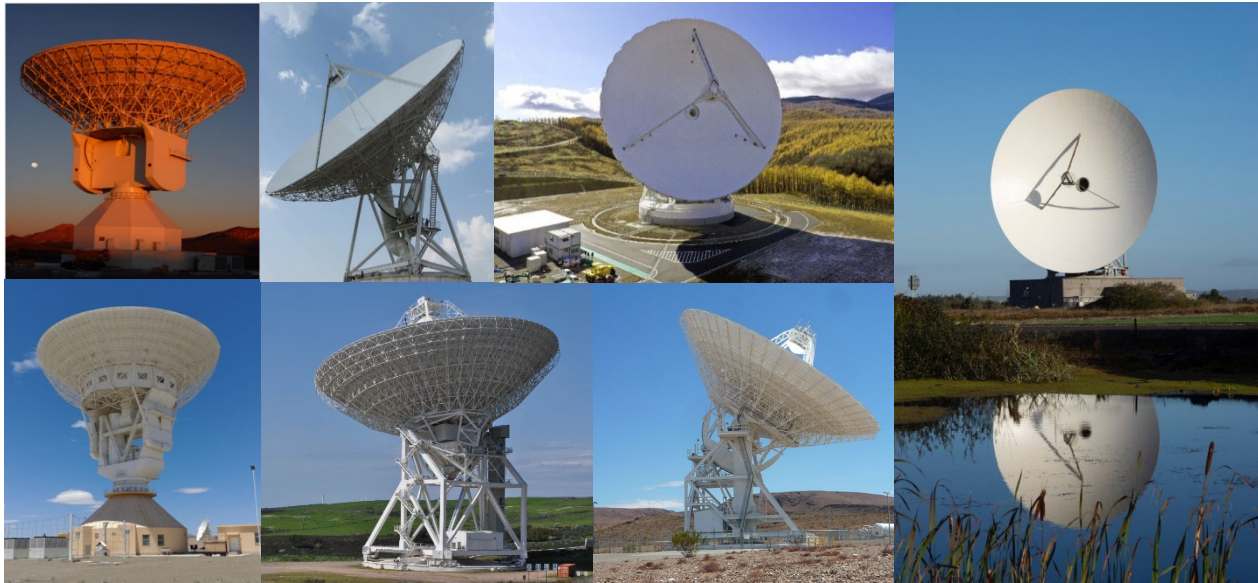
Fig. 1. Ground antennas of IAOG agencies suitable for Mars missions, starting from top left and clockwise: ESA Malargüe 35m antenna, ISRO IDSN-32 antenna, JAXA Misasa 54m antenna, Goonhilly's 32m antenna, NASA DSS-26 34m antenna, ASI-INAF 54m radio telescope/deep space antenna and CNSA Neuquen 35m
